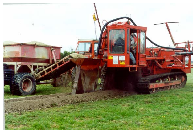
Figure 1. Machine designed for installing subsurface pipes
